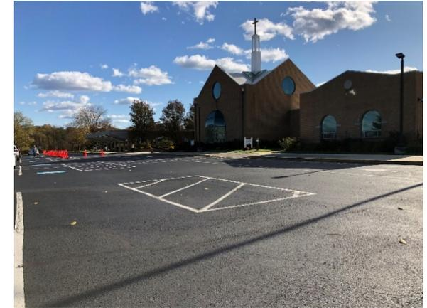
A section of parking spaces can be converted to porous pavement to capture and infiltrate runoff from the rooftop and parking lot. A rain garden can be installed in the turfgrass adjacent to the parking lot to capture, treat, and infiltrate runoff from the parking lot. A preliminary soil assessment suggests that the soils have suitable drainage characteristics for green infrastructure.
